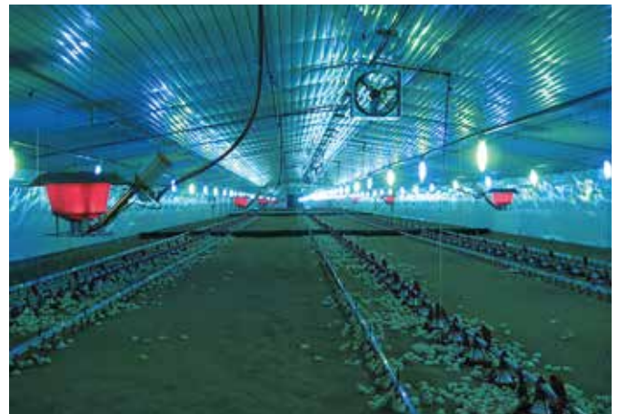
©GASOLEC Orion Green & Blue + G12 Asco G12 Asco heaters in a broiler house. The G12 is known for its wide heat distribution, which comes from a unique reflector design and an emitter which has the largest radiating surface of any 12kW heater. The long lasting G12 is available with either Zone Control or with an Individual Thermostat or Electric Ignition. For information please contact Gasolec B.V. at www.gasolec.com
