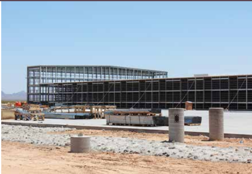
Photo 1 - The construction of a layer barn using the "wrap-in" method (Photo by Author)
